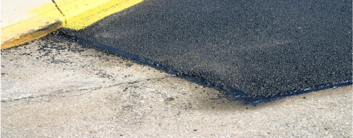
Figure 51 New Asphalt Binder over an Existing Pavement
