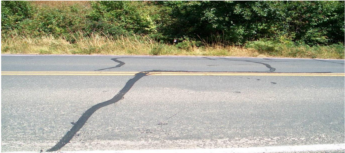
Figure 102 Crack Sealing
