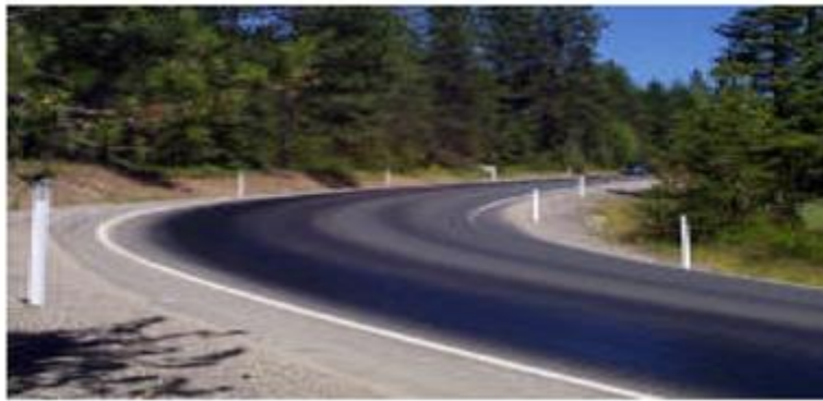
Figure 23 HMA Bleeding from Overasphalting
