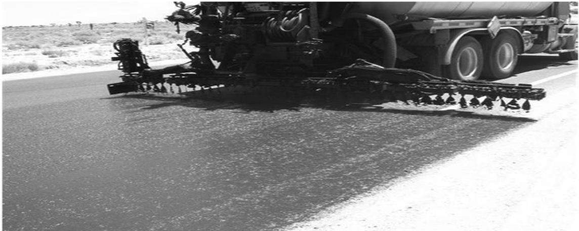
Figure 52 Fog Seal
