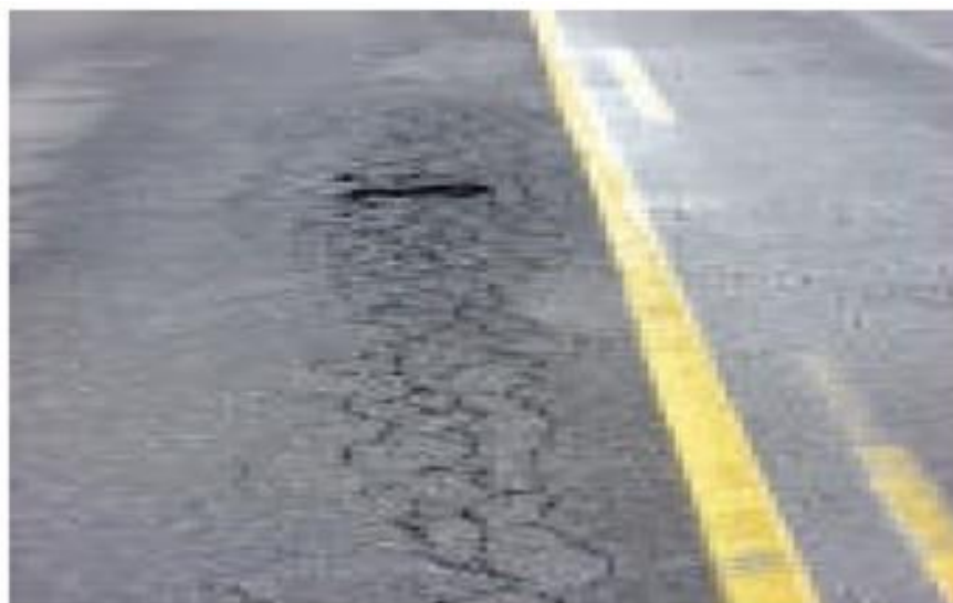
Figure 37 Developing Pothole
