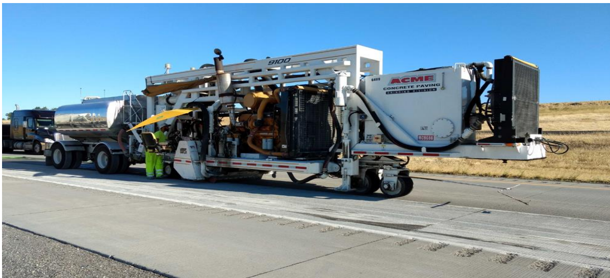
Figure 99 Diamond Grinding
