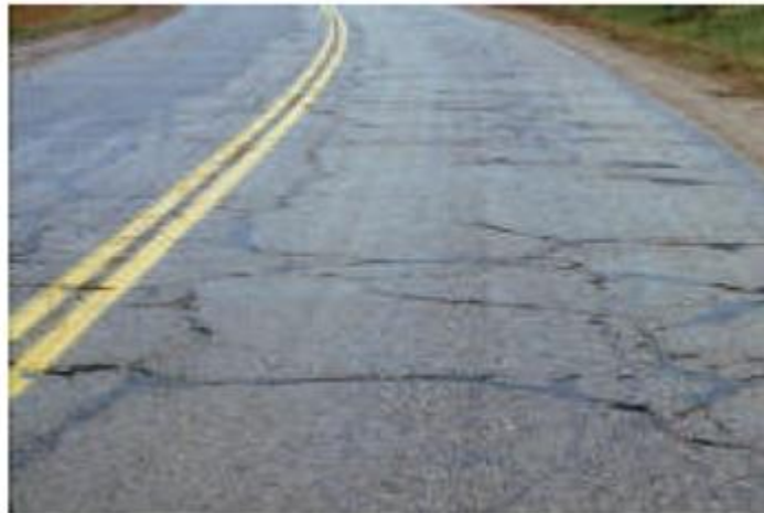
Figure 24 Block Cracking
