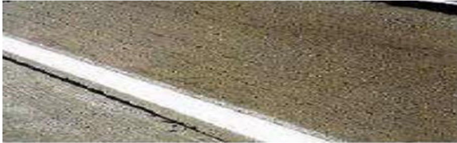
Figure 87 Severe Crazing
