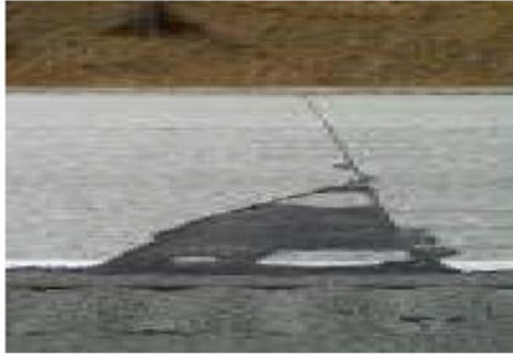
Figure 72 Patched Failure
