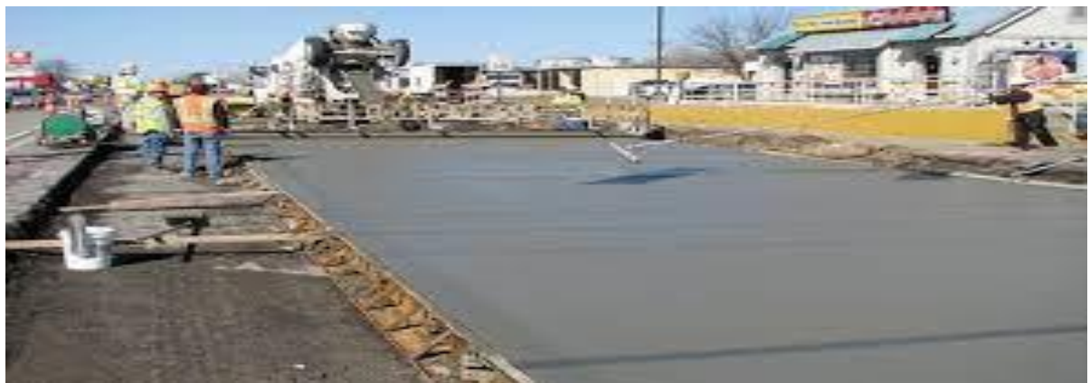
Figure 103 Concrete Overlay
