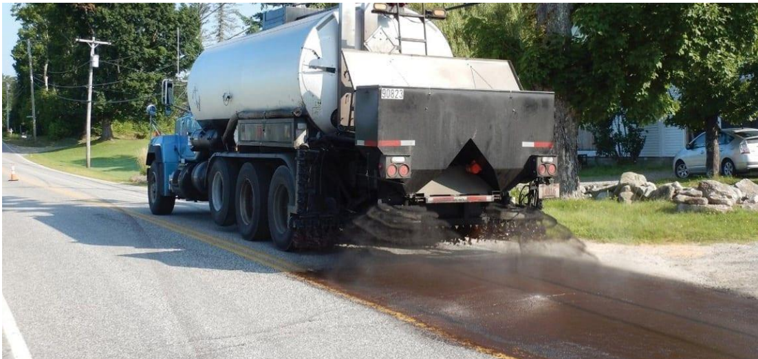
Figure 53 Fog Seal Application
