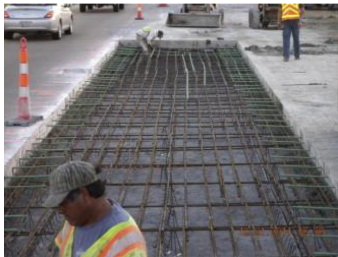
Figure 95 Full Depth Repair
