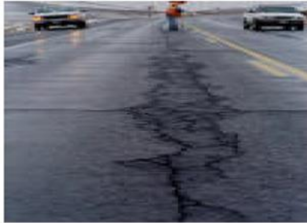
Figure 43 Fatigue Failure from Stripping
