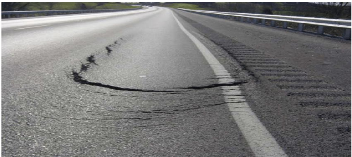
Figure 40 Slippage Cracking
