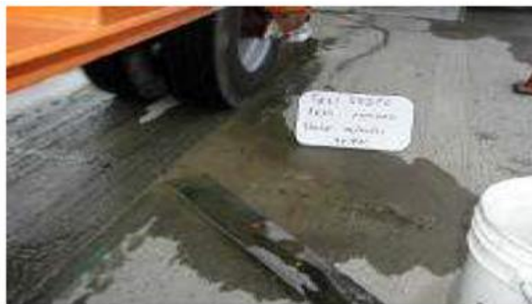
Figure 85 Additional Pumping Evidence during High Vehicle Simulator (HVS) Test
