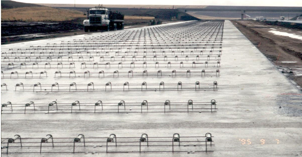
Figure 17 Dowel Bars in Rigid Pavements
