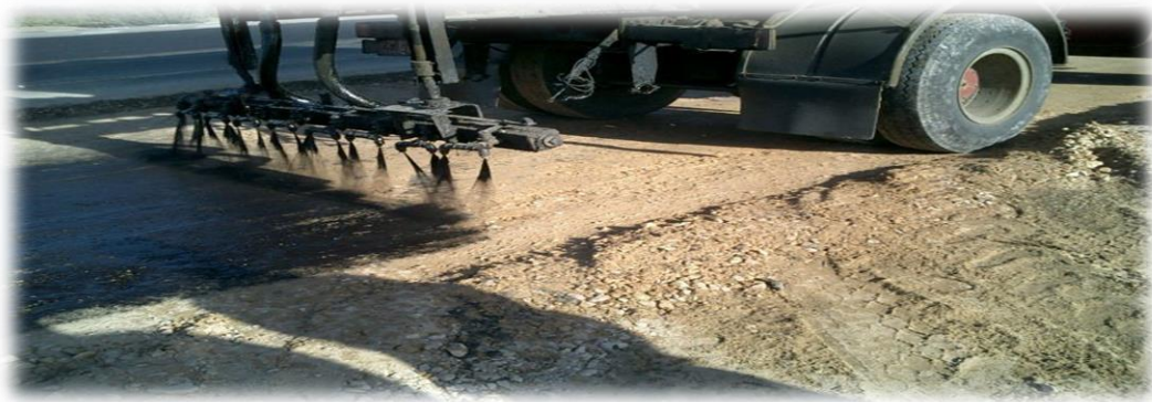
Figure 10 Prime Coat Application
