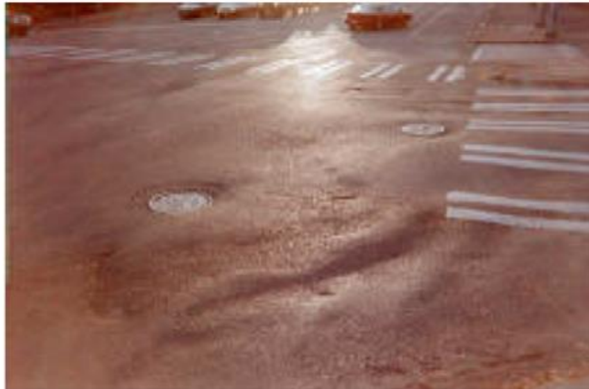
Figure 25 Corrugation and Shoving
