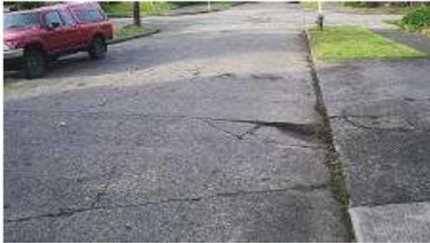
Figure 66 Corner Break on a Residential Street
