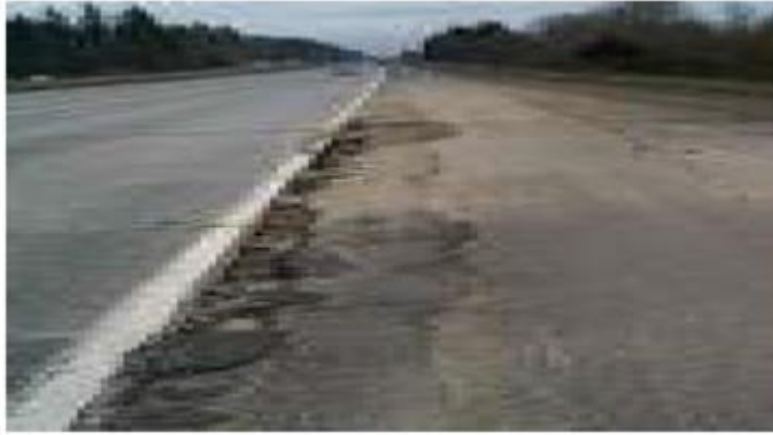
Figure 83 Pumping Damage
