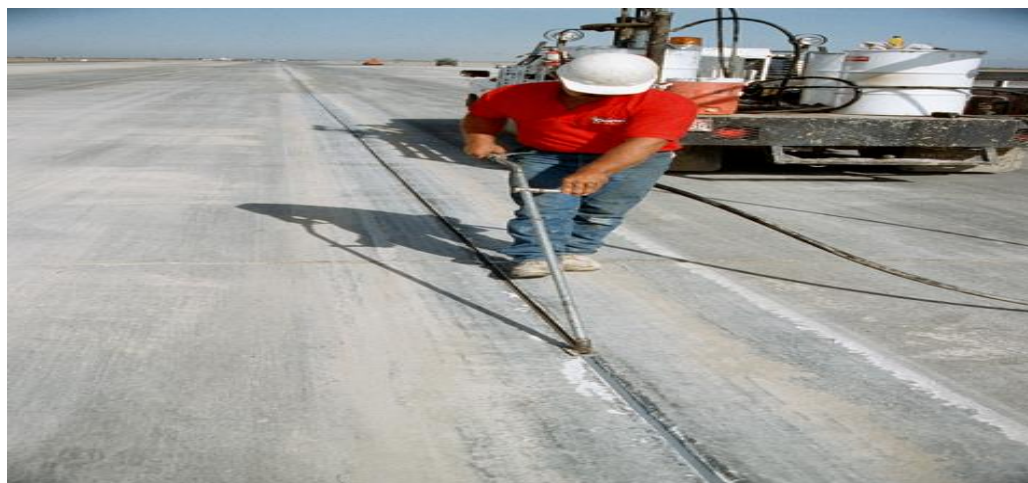
Figure 101 Joint Resealing
