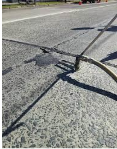
Figure 93 Slab Jacking
