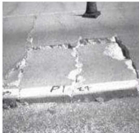
Figure 86 Severe Punchout
