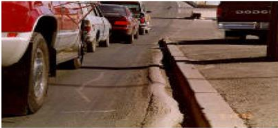
Figure 38 Mix Rutting
