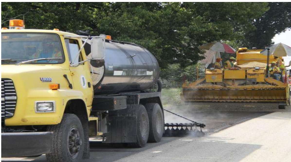
Figure 57 Chip Seal Application
