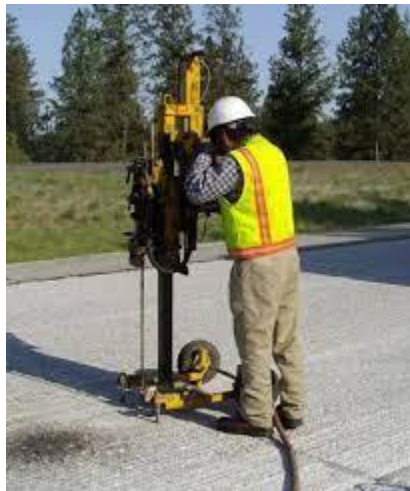
Figure 92 Slab Stabilization
