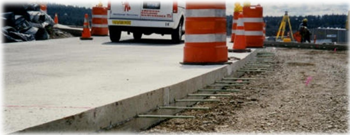
Figure 16 Tie Bars in Rigid Pavements
