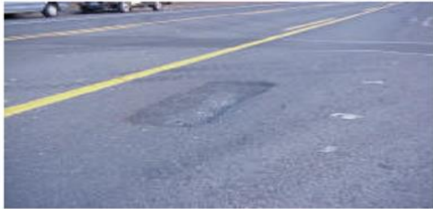
Figure 31 Failing Patch
