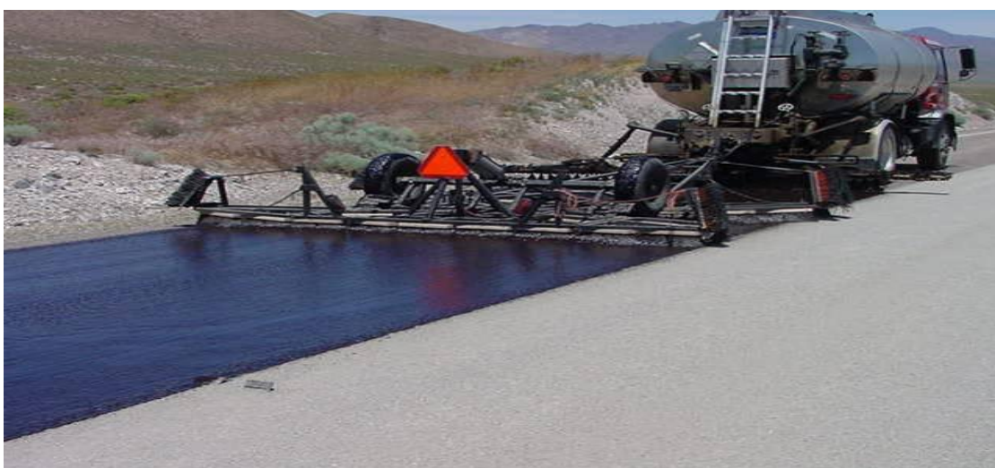
Figure 61 Scrub Seal Application
