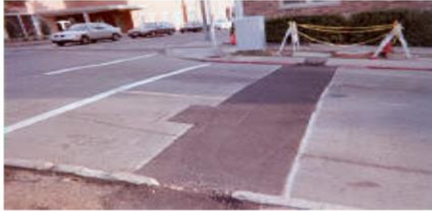
Figure 33 Utility Cut Patch
