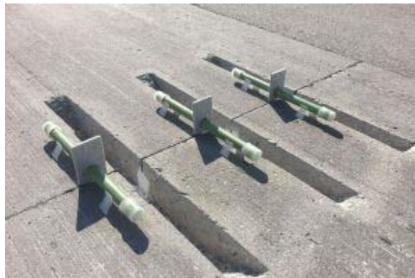
Figure 97 Dowel Bars Retrofit
