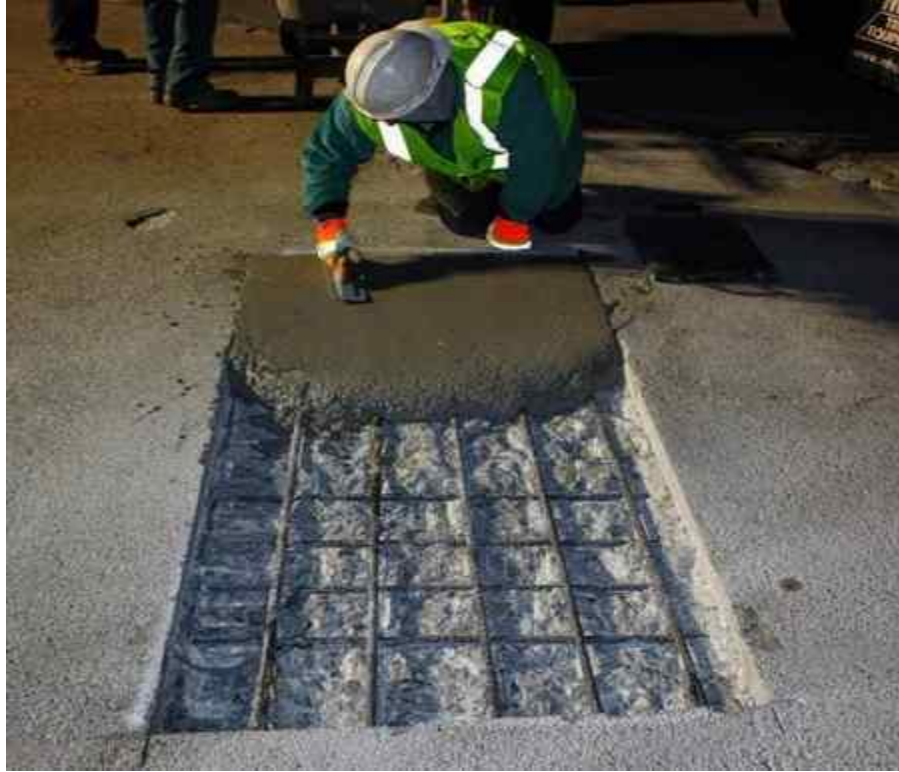
Figure 94 Partial Depth Repair
