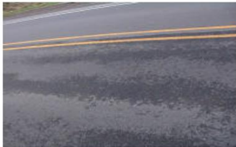
Figure 47 Water Bleeding Up Close
