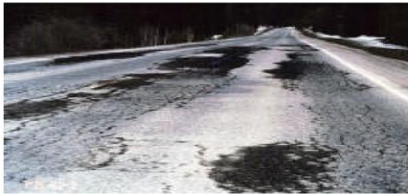
Figure 20 Fatigue Cracking from Frost Action
