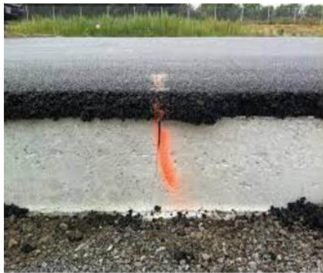
Figure 1 Flexible and Rigid Pavements
