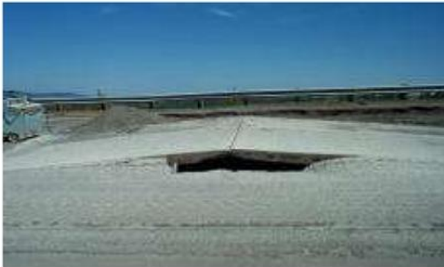
Figure 65 Severe Blowup
