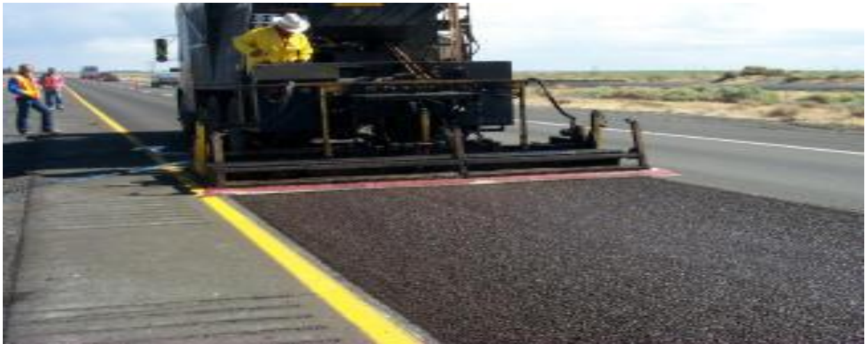
Figure 55 Slurry Seal Application
