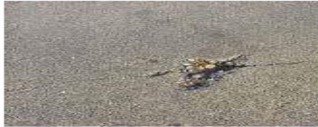
Figure 90 Spalling
