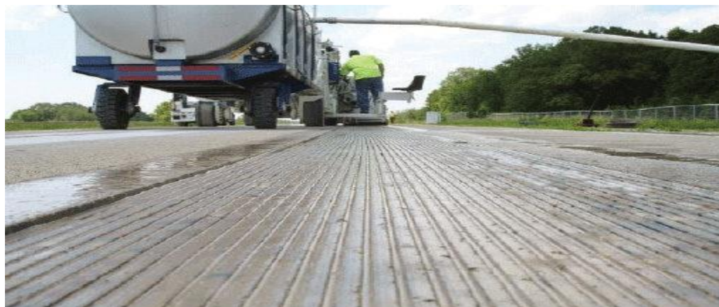
Figure 100 Diamond Grooving
