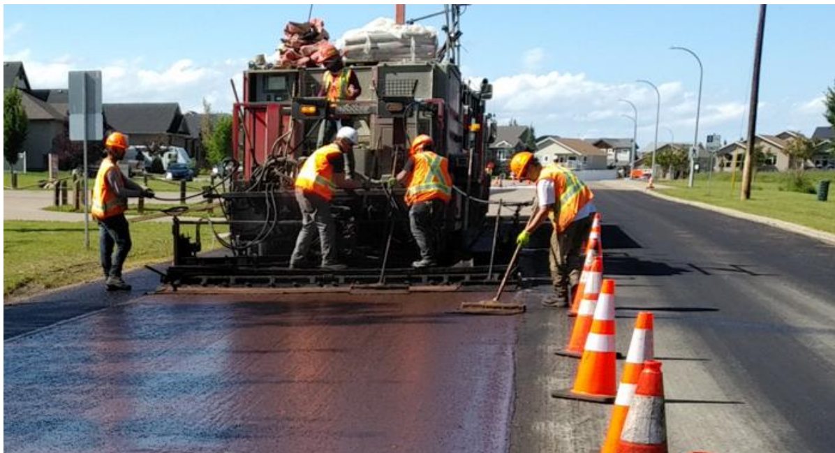
Figure 59 Microsurfacing Application
