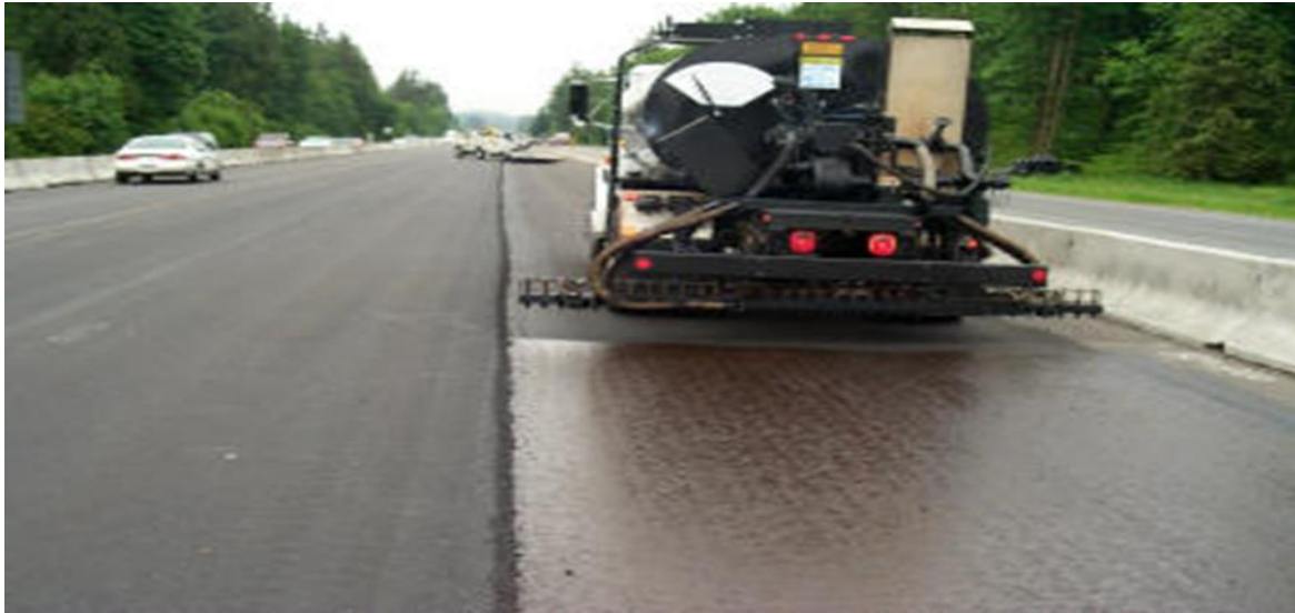
Figure 9 Tack Coat Application
