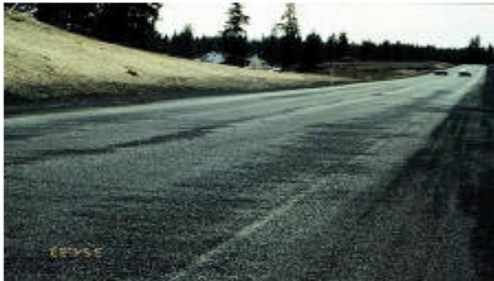
Figure 50 Raveling from Snow Plot
