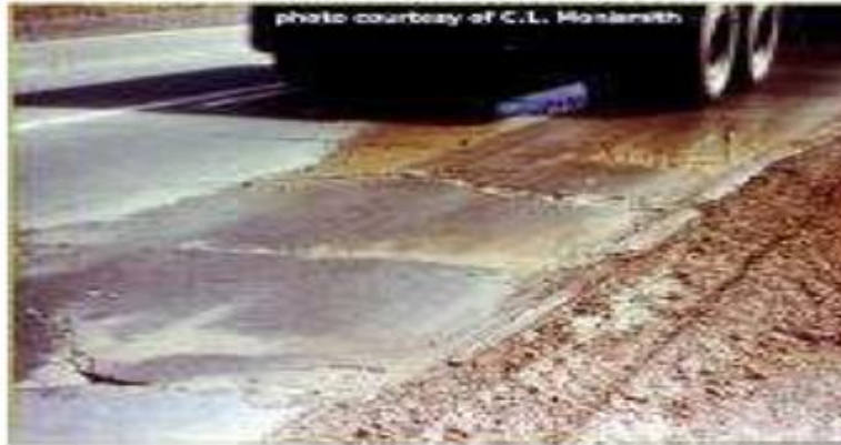
Figure 81 Pumping in Action
